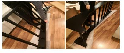
Fit the second rail on the top of the oval bars. Start at one end and progressively insert oval bars until all are seated. Use wooden block and rubber mallet if necessary to fully seat oval bars.
